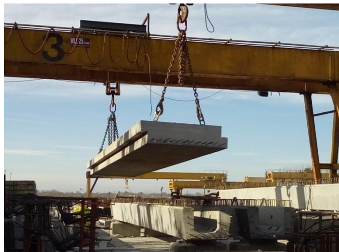
Figure 13. Steel-free pre-stressed beam moving to test rig.
