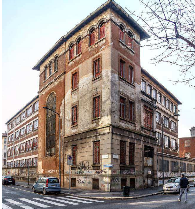
Figure 4. Former Borletti factory building (February 2014, photo taken by Cem Etik during MIAW Workshop, prof. Carlos Arroyo, tutors: E. Fontanella, G. Sempregon, A. Tognon).
