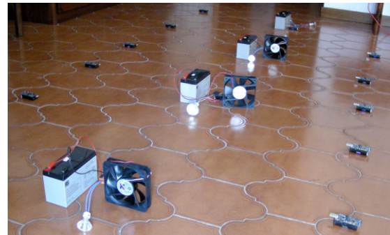
Figure 5. Setup and nodes controlling fans and lights.
