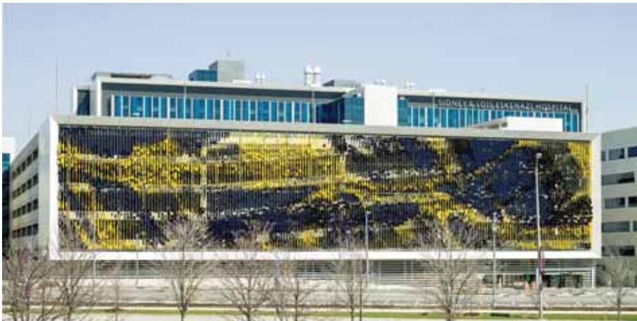
Fig. 4 - Parking Structure Art Façade, Indianapolis, IN, USA (2014) by Urbana Studio (Rob Ley). Photo © Serge Hoeltzsch.
