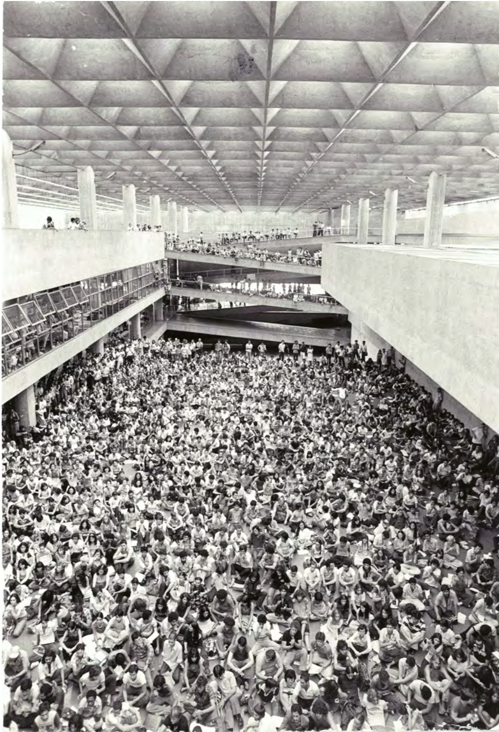
→ J. B. Vilanova Artigas, FAU, São Paulo, 1961-69, view of the big court during a meeting of students © Raul Garcez © Acervo João Batista Vilanova Artigas / FAUUSP.
