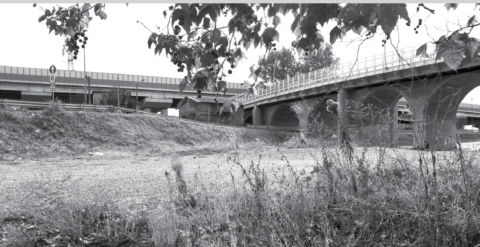
Pò riverbank and infrastructure - photo by Filippo Orsini
