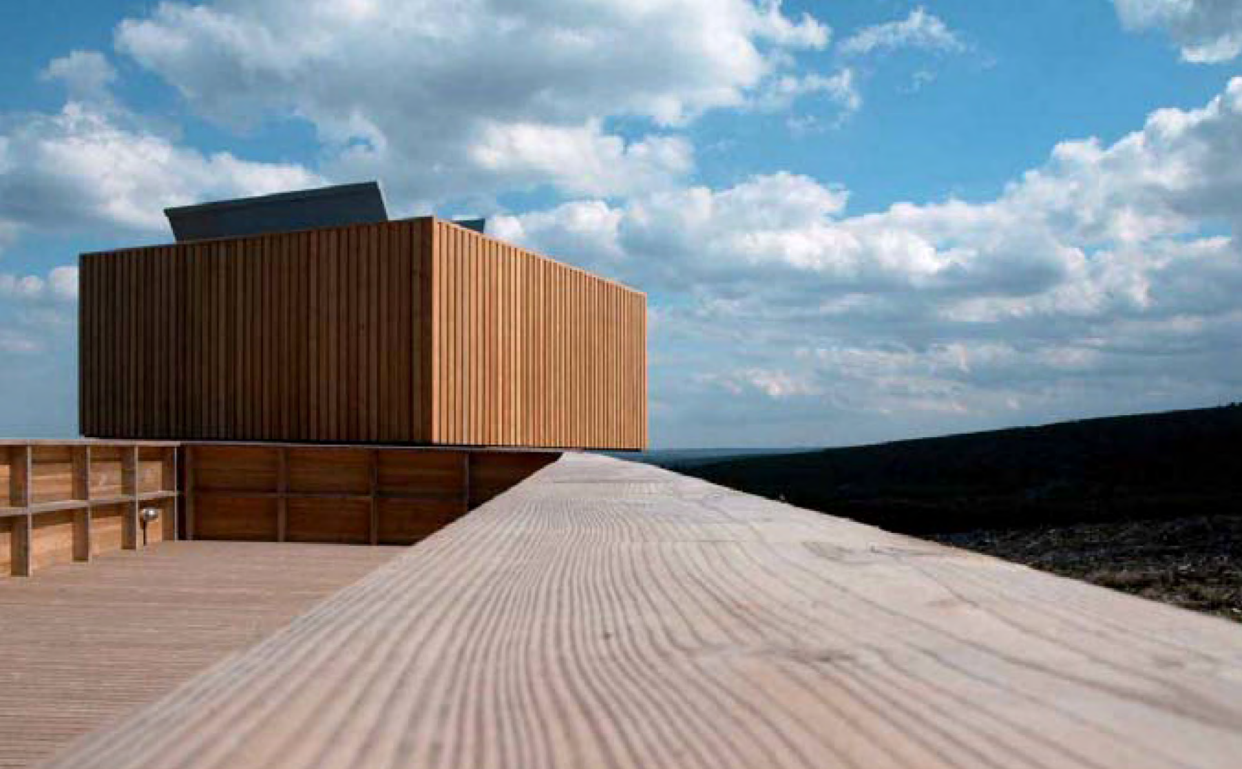
Observatoire Kielder , Charles Barclay Architects, Northumberland, Angleterre, 2008.
