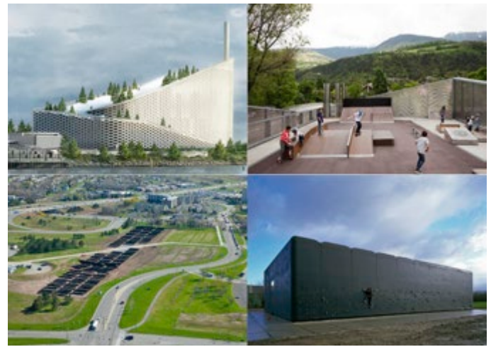
06 | Approccio integrato (multifunzionalità): da dx in alto, senso orario: Modus Architects - Centrale di Cogenerazione e skate park, Bressanone (BZ), 2007 (© Paolo Riolzi), NL Architects, WOS 8 Heat Transfer Station, Utrecht, Olanda (fonte: www.nlarchitects.nl ), Hood Design, Solar Strand, Buffalo, Stati Uniti, 2012 (fonte: www.buffalo.edu ), BIG, Termovalorizzatore e pista da sci Amager Bakke, Copenhagen, Danimarca, in costruzione (fonte: http://www.dwell.com ) Integrated multifunctional approach: clockwise from top right: Modus Architects - Cogeneration plant and skate park, Brixen (BZ), 2007 (© Paolo Riolzi), NL Architects, WOS 8 Heat Transfer Station, Utrecht, NL (source: www.nlarchitects.nl ), Hood Design, Solar Strand, Buffalo, USA, 2012 (source: www.buffalo.edu ), BIG, Amager Bakke Waste to energy plant and ski slope, Copenhagen, Denmark, under construction (source: http://www.dwell.com )
