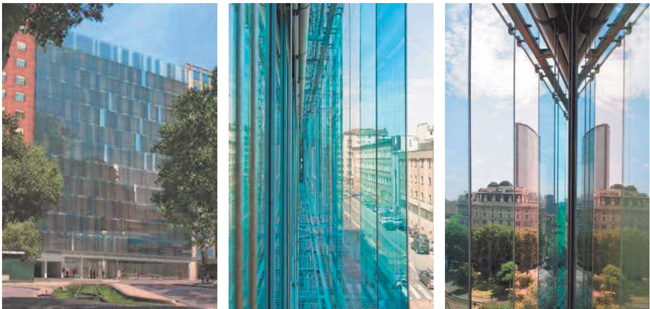
Figures 8-9-10: some images of the double skin building envelope of the Blend Building.
