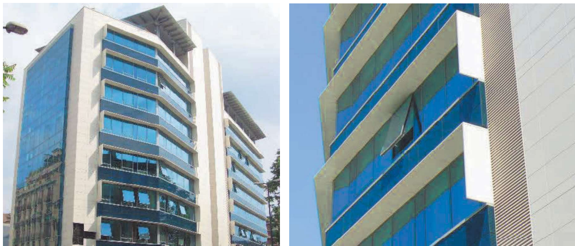
Figures 4-5: On the left, the ventilated façade and structural curtain wall; on the right, a detail of the ventilated facade.
