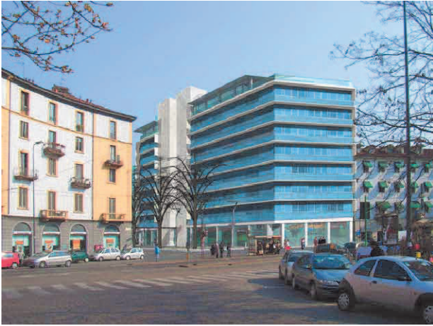
Fig. 4 The property in via Vespucci after the re-development operation to the building envelope. (Source: General Planning).
