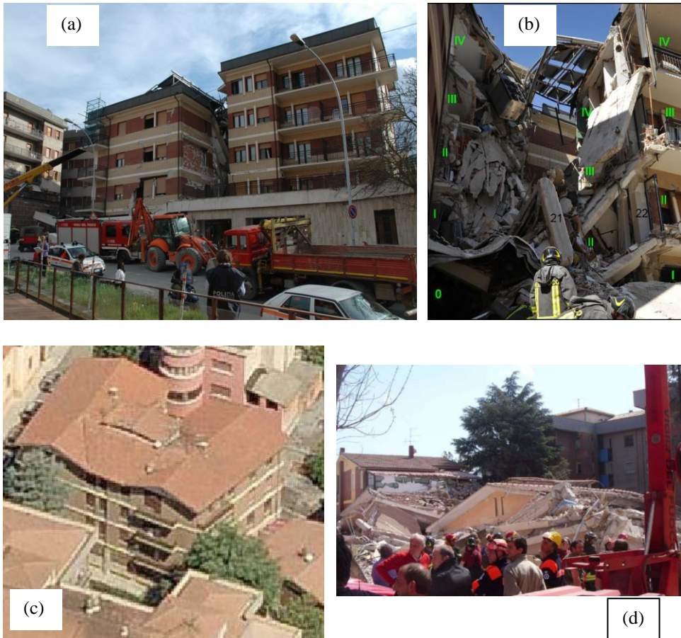
Figure 1: “Casa dello studente”, (a-b) soft-storey of the North wing. Via D’Annunzio, (c-d) before and after the earthquake.
