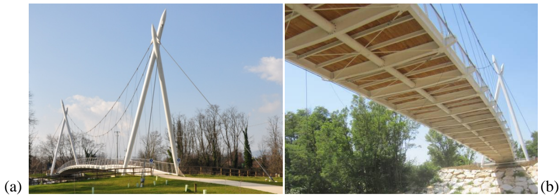
Figure 1. Seriate Footbridge: (a) overall view; (b) footbridge deck, detail of longitudinal and transverse beam.
