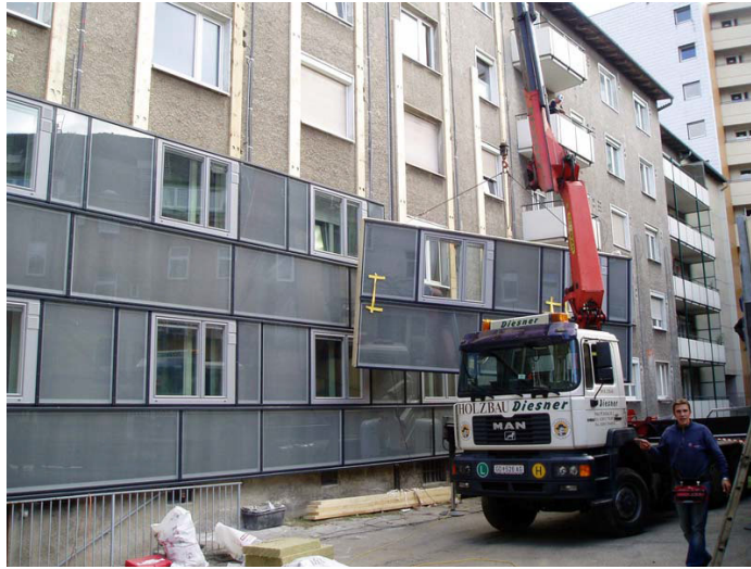
Fig. 2 Installation of the panel in Makartstrasse, Linz (Germany)
