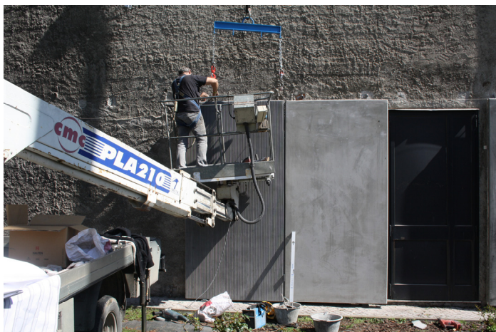
Fig. 3 Installation of EASEE panels
