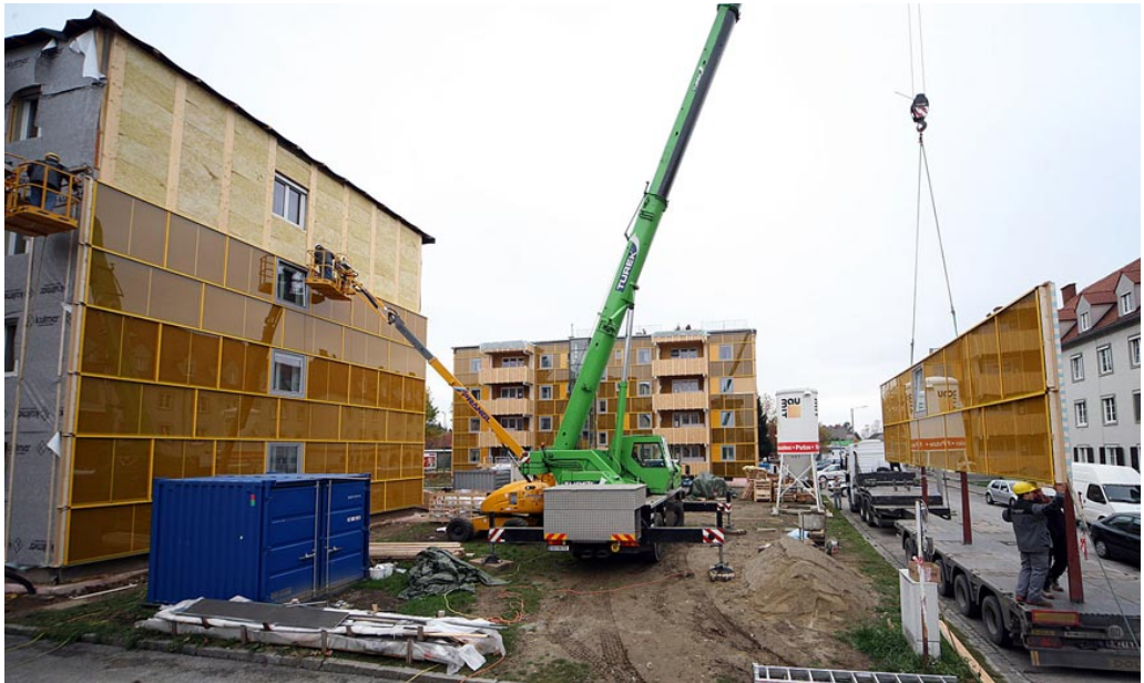
Fig. 1 Installation of the large panels in Dieselweg, Graz, Austria
