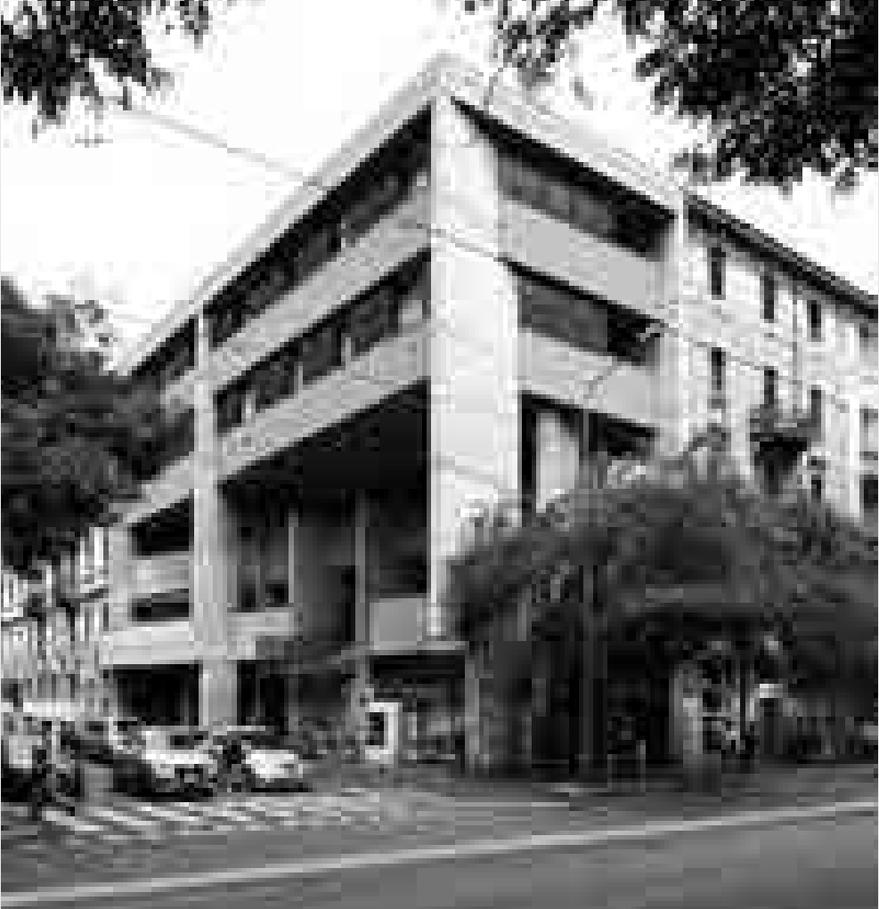
The brutalist corner on Corso XXII Marzo interrupting the XIX century façades.
