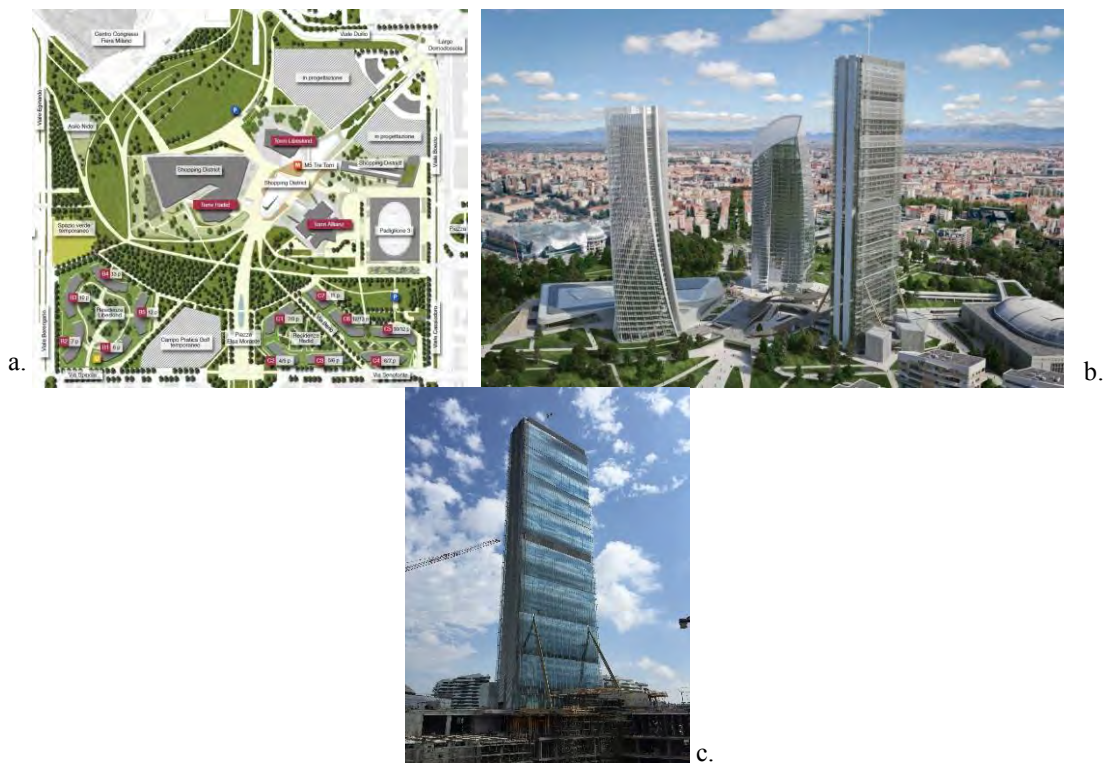
Fig.1 – a. Masterplan of the CityLife Development; b. Architectural rendering of the three CityLife Towers (Allianz Tower is on the right), c. The topped-out Allianz Tower
