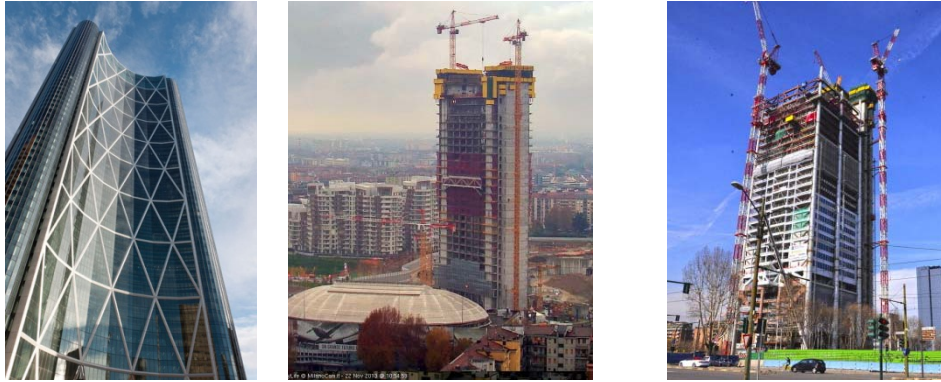
Figure 1: a) Tall building shear restraint core and steel frame b) Concrete frames with large steel elements c) Steel frames collaborating with shear resisting concrete cores
