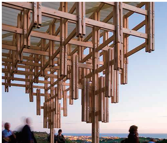
Fig. 5: Traditional Japanese bracket system and its reinterpretation.
