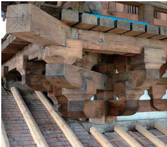
Fig. 5: Traditional Japanese bracket system and its reinterpretation.
