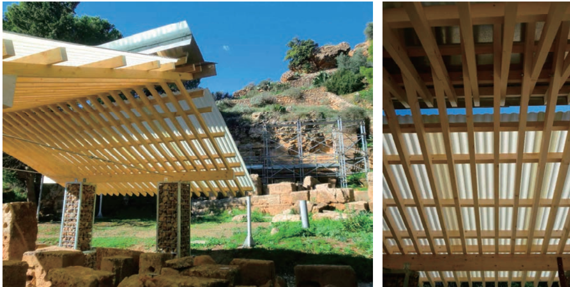
Fig. 2: The shelter sits by a temple dedicated to Demeter, wife of Zeus. Fig. 3: Detail of the roof.
