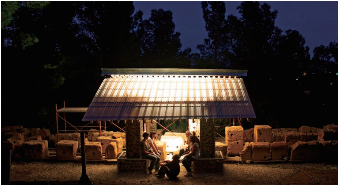
Fig. 1: White corrugated fiberglass covers the shelter giving it a soft atmosphere.
