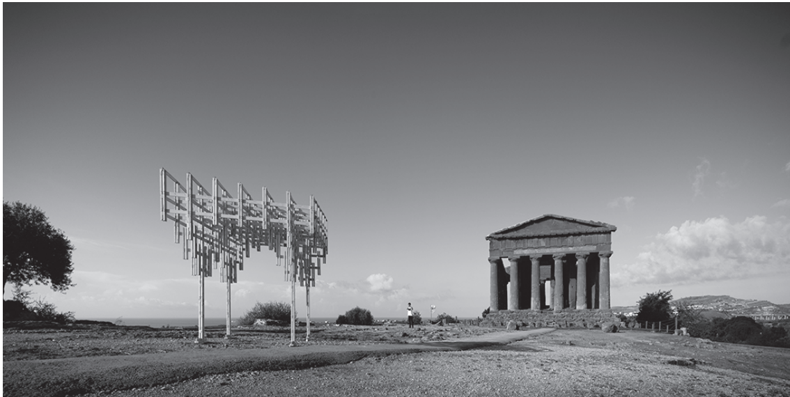
Fig. 4: The shelter integrated in the Valle dei Templi, close to the Temple of Concordia
