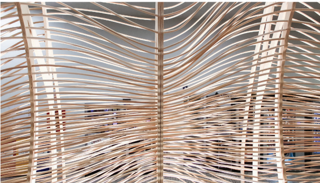
Figure 19: The variable density of rattan wefts generates a differential screening ratio along Weaving Enclosure surfaces.
