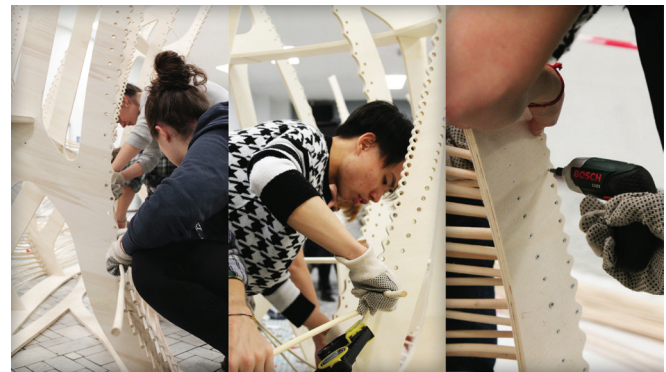
Figure 17: Manual work is still a fundamental step in the weaving process. Right. Screwing process for rattan post-tensioning.
