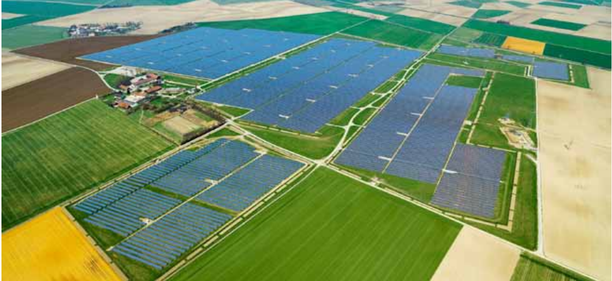
Open field photovoltaic installation in Germany
