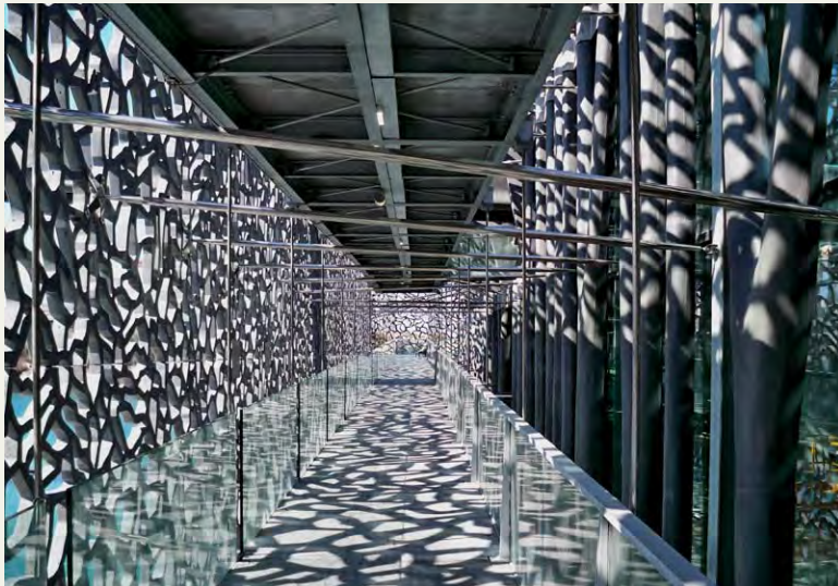
IMG. 3.76 — View of the ramp that goes up from ground floor to the terrace. A public path connects the museum and the fort and, using a similar footbridge, the fort and the Panier district. Photo by Luca Basso Peressut.
