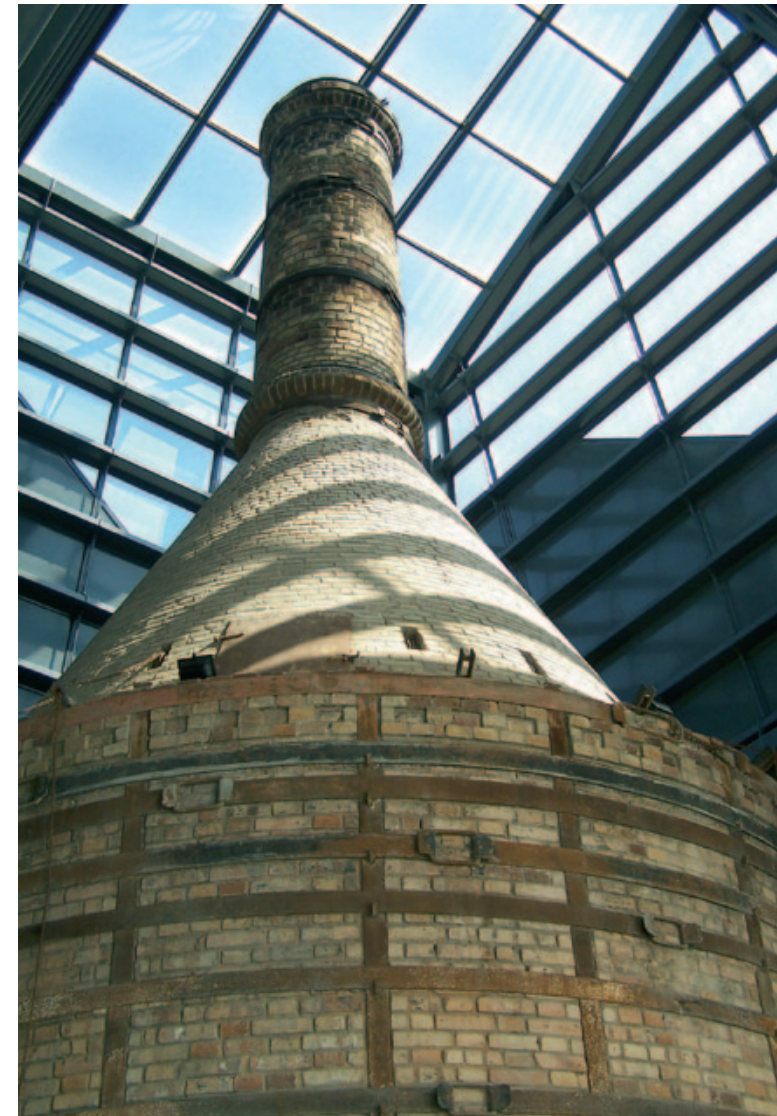
IMG. 6.16 — Museu de Cerâmica, Sacavém, Portugal. The number 18 furnace of the old faience factory. Photo by Filipe Rocha.
