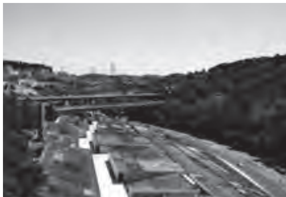
João Nunes, ETAR Water Treatment , Lisboa, 2005-11
