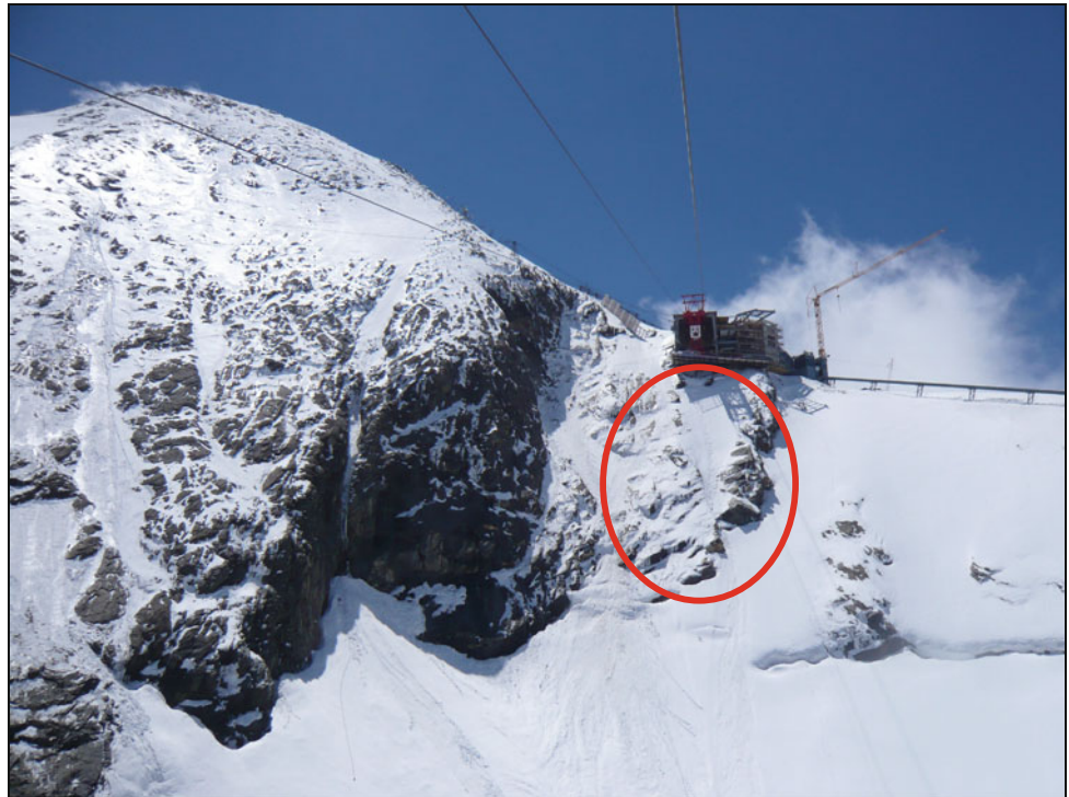
Fig. 56.1 Overview of the project area on the Kitzsteinhorn (view towards South)
