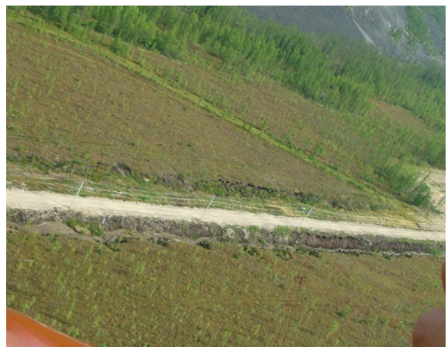
Fig. 58.3 Dangerous site with thermoerosion on the polygons with ice wedges along oil pipeline "Eastern Siberia–Pacific Ocean-1" (ESPO-1) in Chulman area
