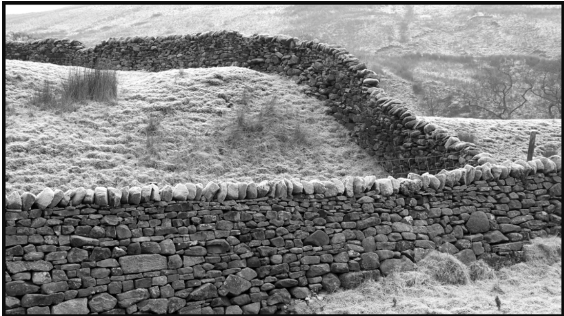
Fig. 6 Dry stone walls
