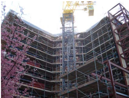
Fig. 6: Uxbridge Travel Lodge Hotel, a cheaper and faster construction built with 86 shipping containers, in west London, United Kingdom. Photograph by Lara L. Barbosa.
