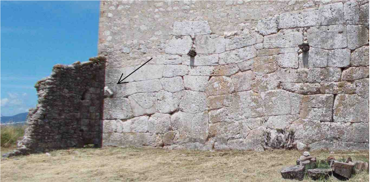
Fig. 6. Grotte di Torri in Sabina (Rieti). The north-west corner of the polygonal walls seen from the west, with the corner block with reliefs evidenced by an arrow. The remains of an orthogonal wall of small stones come from a later addition. (Photograph G. Magli)
