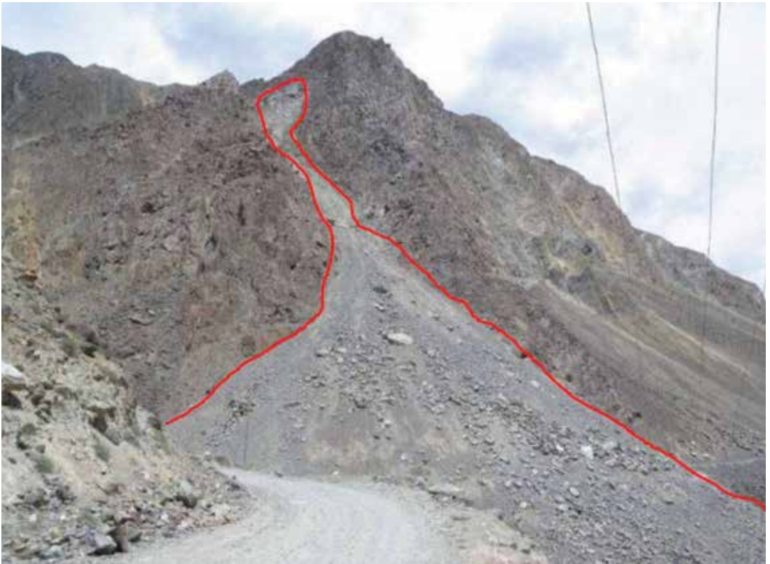
Fig. 5. Landslide in Bagrot valley.
