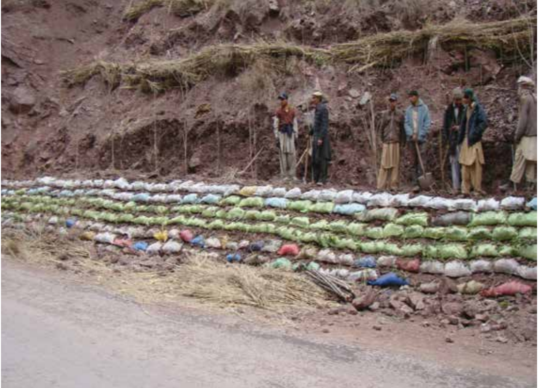
Fig. 12. Example of bioengineering structure for landslide containment.
