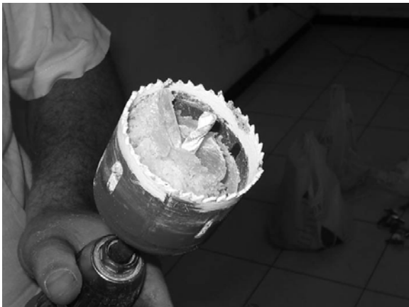
Figures 9-10. Coring of the wallboard.
