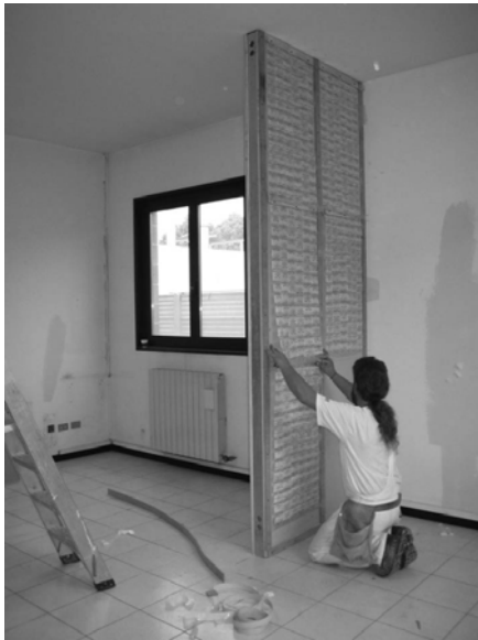
Figure 3. The installation of the blanket.
