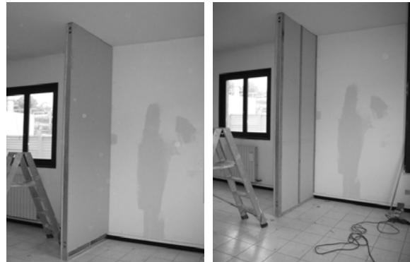
Figures 6-7. Application of PCM blanket.
