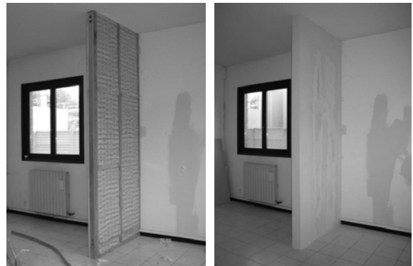
Figures 7-8. Outer layer boarding and finishing.
