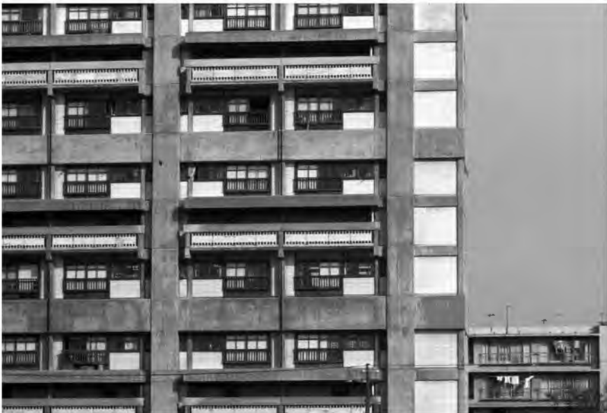
Figure 7.1 Kunio Maekawa, Harumi Apartments, Tokyo, 1957.
