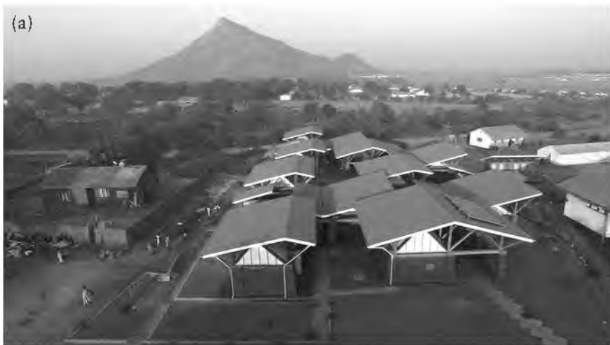
Figure 6.4 (a) MASS Design Group, Maternity Waiting Village, Kasungu, Malawi, 2015. Birds eye view. (b) View from above of the open air space. (Continued)
