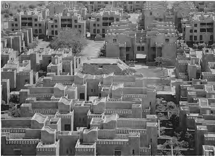
Figure 4.3 Raj Rewal, Asian Games Village, New Delhi, 1982. (a) Bird's-eye view. (b) Detail of housing block.
