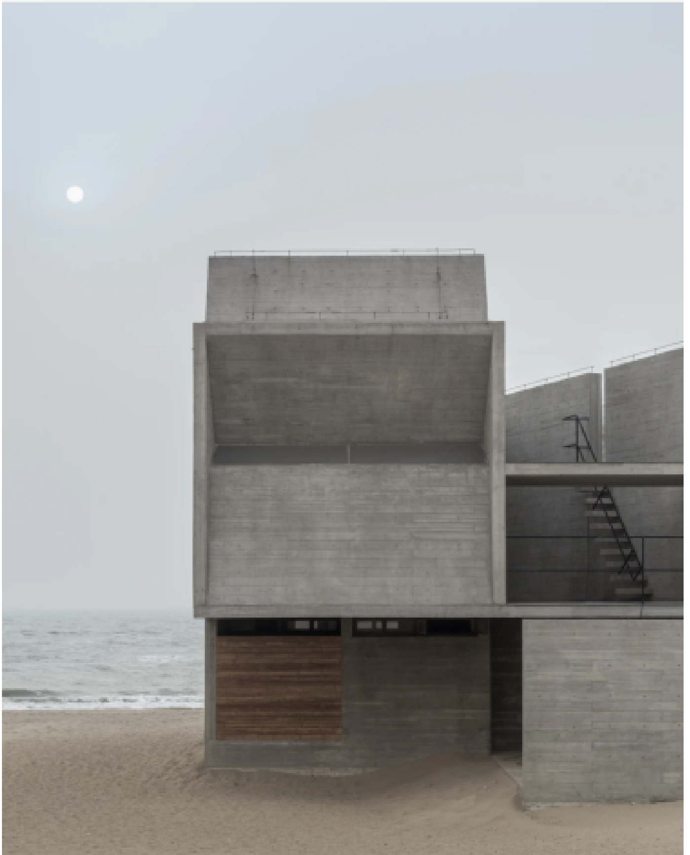
Figure 2. The Seashore Library, Vector Architects – Credit: James Florio
