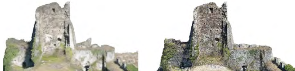
Figure 20. Point clouds produced with Nerfstudio ( left ) and Metashape ( right ) using the same set of images for the Vogogna dataset.
