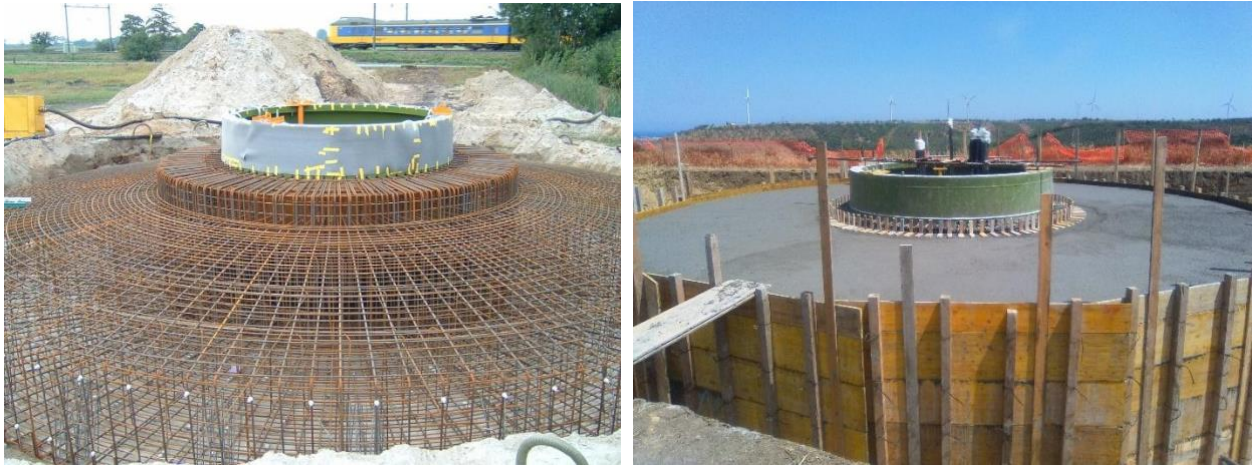
8 9 Figure 2. Example of concrete foundation for onshore steel turbine: reinforcement rebar 10 arrangement (left) and concrete block (right).
