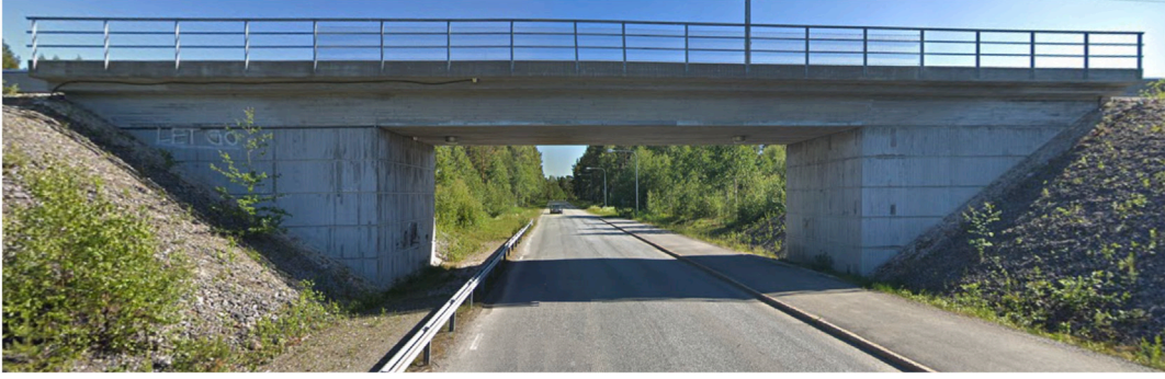
Fig. 9. Hörnefors railway bridge.
