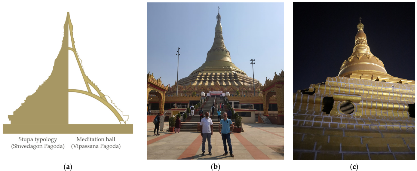
Figure 1. (a) Scheme comparing the cross-sections of a traditional Burmese stupa and the Global Vipassana Pagoda typology. (b) General outer view of the Global Vipassana Pagoda with one of the authors and (c) particular of the external skin.
