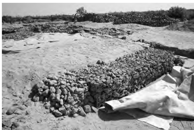
Fig. 26 - Sector 6, Cathedral: South wall, consolidation with stone box.
