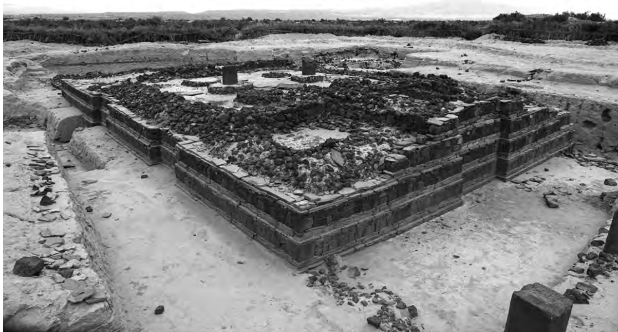
Fig. 7 - Northern Urban Church: general view from south-east of the podium with recesses.
