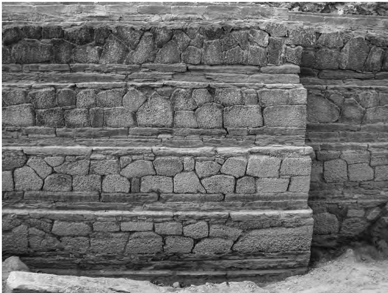
Fig. 4 - Northern urban Church: Construction Techniques.
