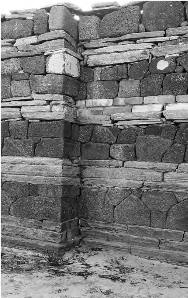
Fig. 21 - Northern Urban Church. Preservation intervention: reconstruction of a necessary new structural part with schist and basalt (altar retaining wall, east side) clearly evident with the insertion of a different material: a brick course that indicates the intervention.
