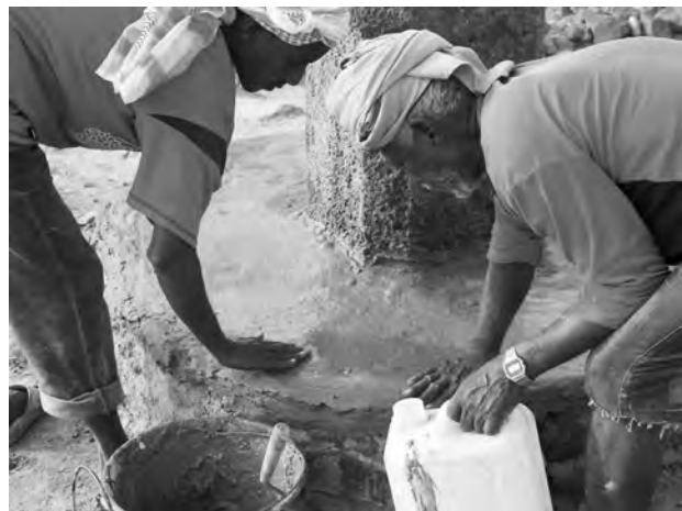
Fig. 23 - Sector 2, Northern Urban Church. Preservation: waterproofing for exposed surfaces with ‘ cicca ’, a traditional organic mortar consisting of clay, animal hair, and manure.
