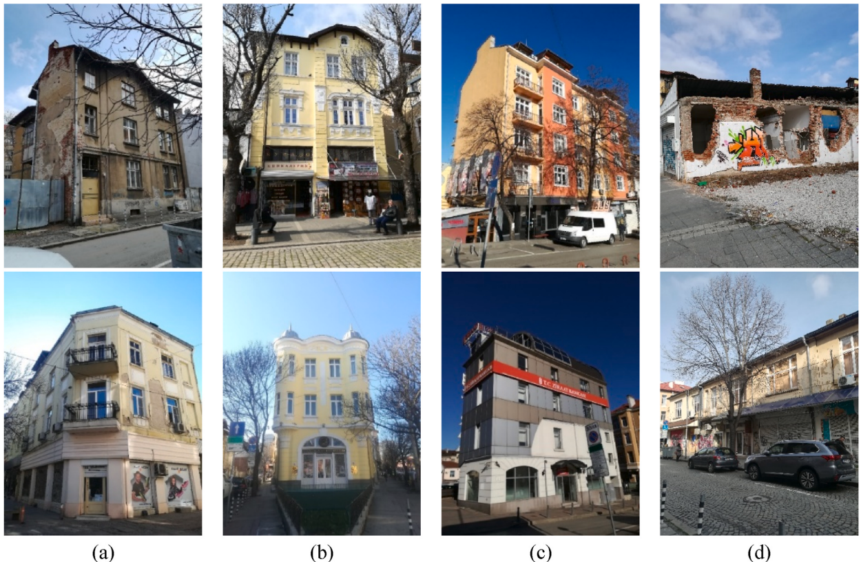
Fig. 2. Building typologies of the C01 sector: masonry buildings with steel beam floors with brick infill (a), masonry buildings with reinforced concrete floors (b), reinforcing concrete buildings (c) and disused buildings (d).
