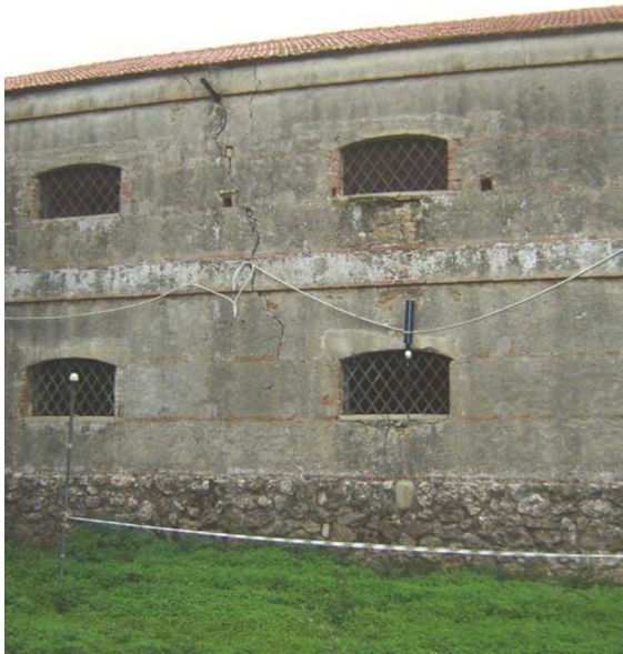
Fig. 3 North-wall of the structure. Image taken from [59]
