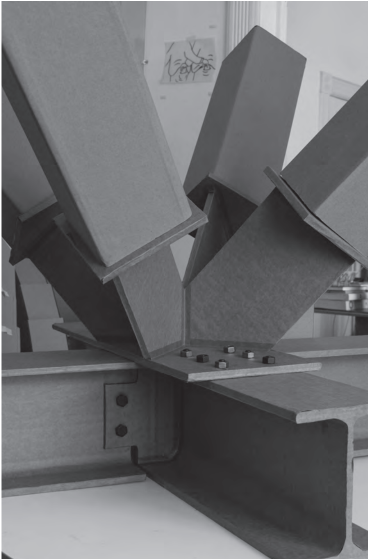
Suspended house w/Productora, 1:1 scale model beam connection (7); © Taller Isidoro Michan-Guindi.
