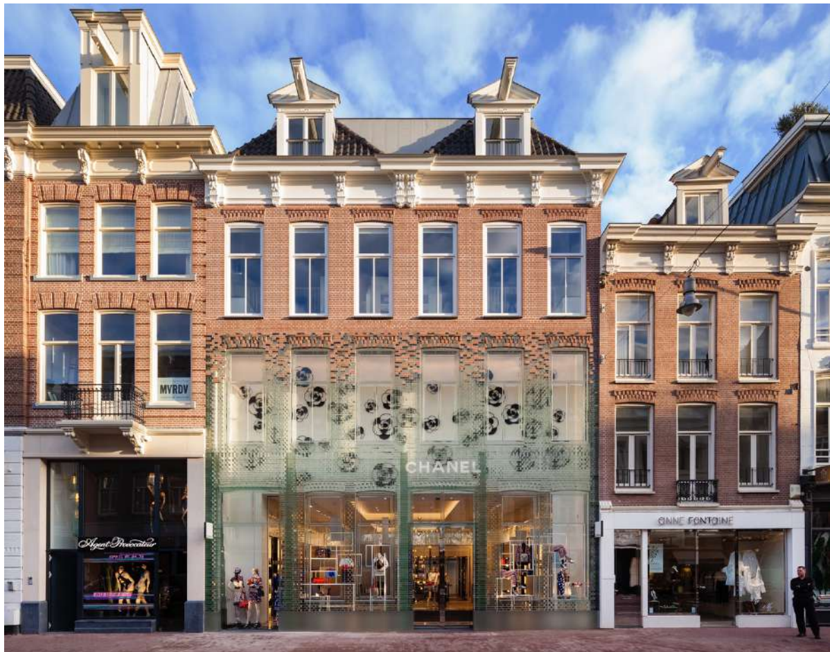
Figure 1 The facade shows the fading of glass brick and its transition to traditional brick
