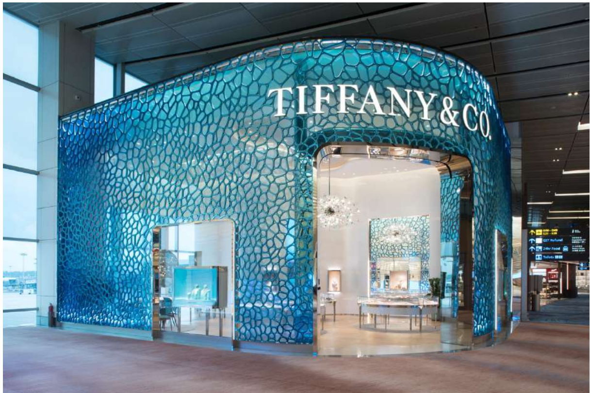
Figure 7 The 3D-printed screen of the facade
