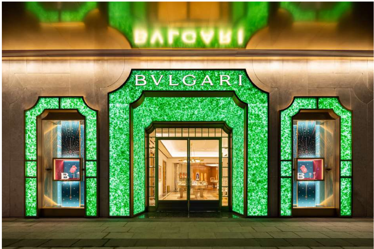
Figure 5 Art deco-inspired profiles of façade openings
