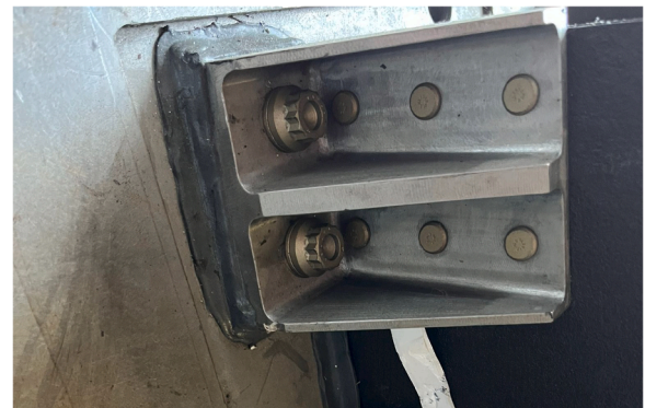
Fig. 19. Detail of the mechanical connection bracket-stabilizer (rivets) and bracket-steel plate (bolts).
