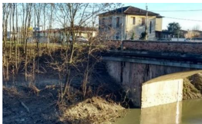
Figure 3. Survey site conditions in the preliminary inspection.
