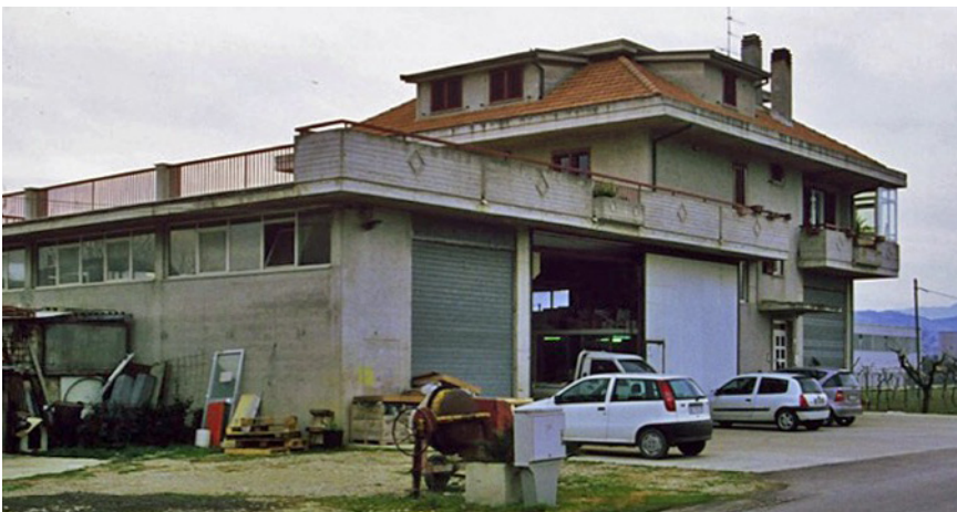
Fig. 26: Family house and working shed, Valle del Tronto, Marche region, late 1990s; photographer: Chiara Merlini
