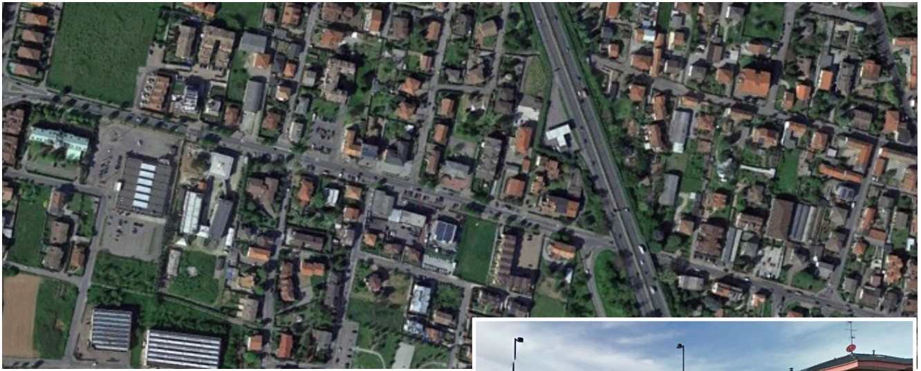
Fig. 30a (above): Conurbated settlements of family houses and amenities along a Provincial road between Seveso and 30b (right): Seregno, Lombardy region; source: Google Earth, 2014
