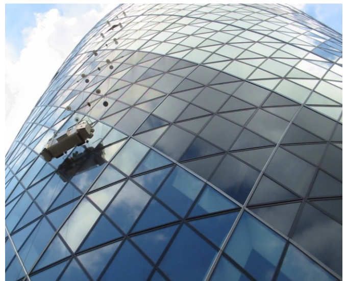
Fig. 2 Norman Foster and Partners, Swiss Re Tower, London. Type of enclosure enveloping the cylindrical tower, streamlined and tapered according to a progressive double-curved conical winding. The enclosure, warped by the diagonal lattice construction, is composed of the double envelope system that generates an upward air flow (stimulated by the “chimney effect” and increased by the thermal gradient between the temperature in the cavity and the temperature of the incoming air) © by the Author
