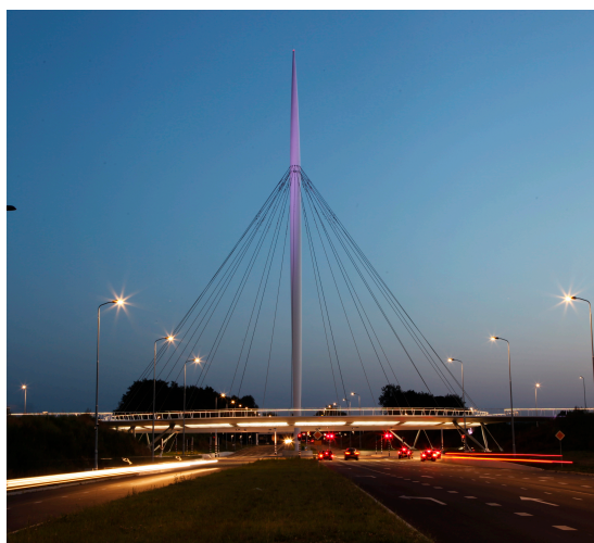
(a) The bridge
