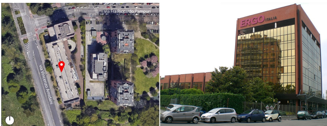
Figure 2. Plan and street view of the case study building in the pre-retrofit status.
