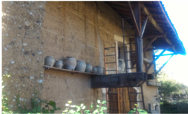
Figure 1: Rammed earth house in the village of St. Chef, Iserre, south of France.
