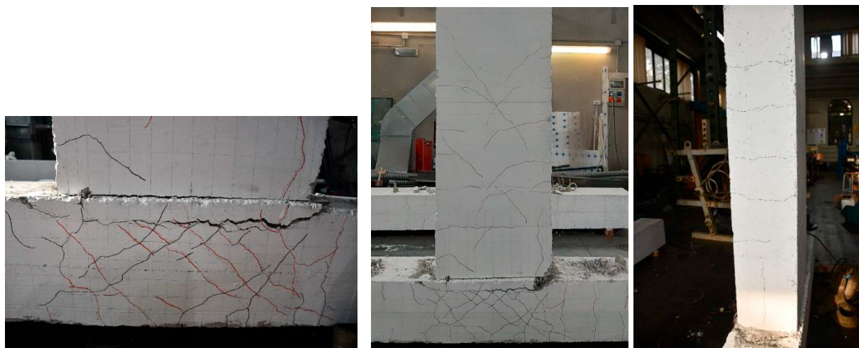
Fig. 9. Specimen BCJB after failure.
