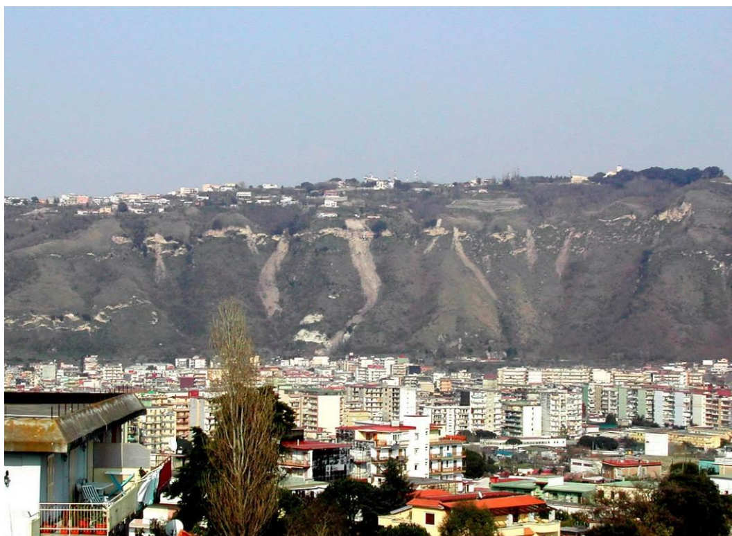
Figure 1. Landslides occurred on the 4th and 5th of March 2005 along the western slope of Camaldoli Hill facing the Pianura borough of Naples.
