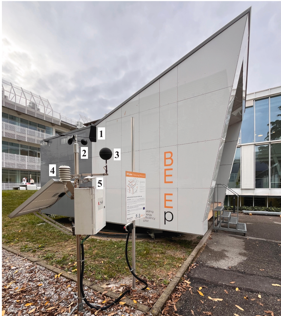
Fig. 1. Weather station installed nearby the testing facility and equipped with: wind direction sensor (1), anemometer (2), globe temperature sensor (3), air temperature and relative humidity sensor (4), class A pyranometer (5).
