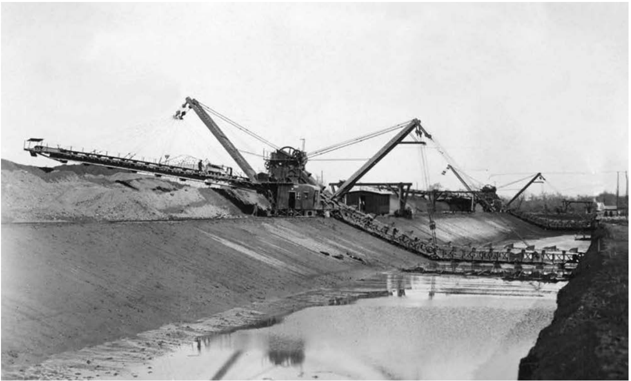
Fig. 2 Excavators at Casale Perazzotti, Acque Alte channel, near Latina, in 1929 (from Zucaro 2012).
