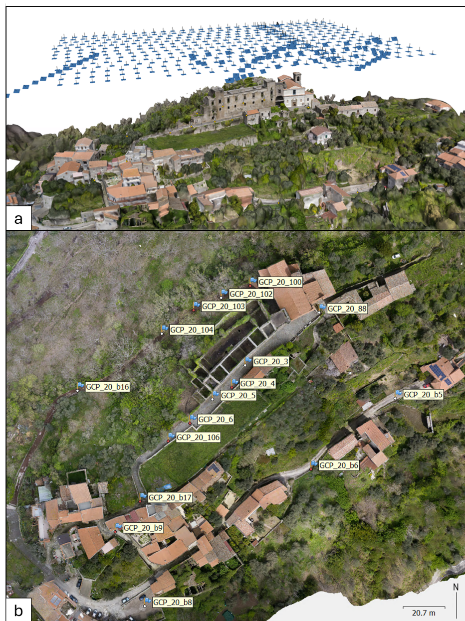
Figure 6. (a) The dataset used for scenario I. In this image, the mesh model is visible on top of the image; it is possible to see the camera locations. (b) The GCPs and CPs used throughout the tests performed within scenario I, positioned around the castle area.
