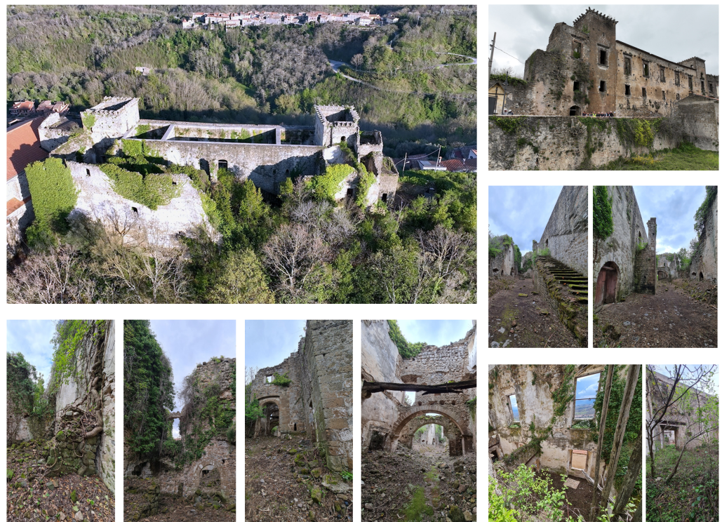
Figure 2. Pictures of the Castle of Terracorpo in its actual status.
