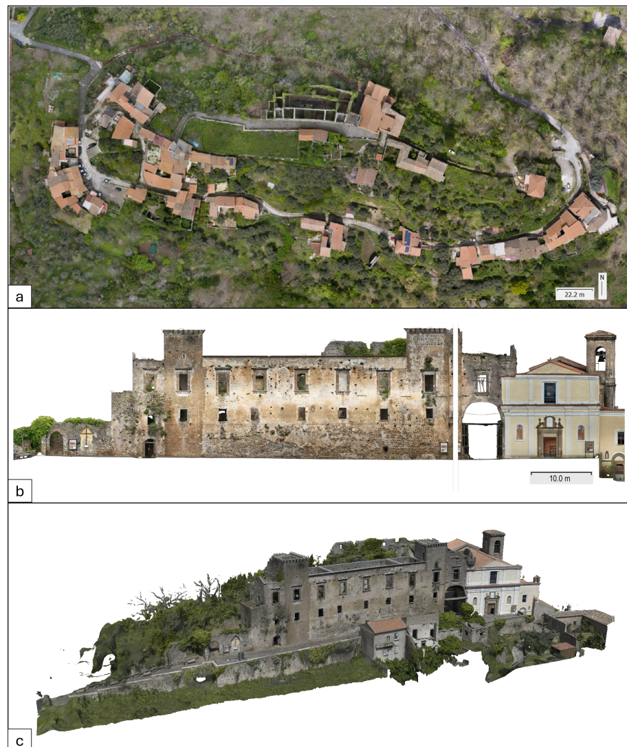
Figure 12. Examples of deliverables obtained through the photogrammetric process in the case study exploiting UAV data. (a) Orthophoto of the castle and its surroundings. (b) Orthophoto of the facade of the castle. (c) Three-dimensional model (texturised mesh) of the castle.
